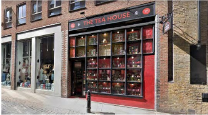
15A, Neal Street – Existing West Façade
