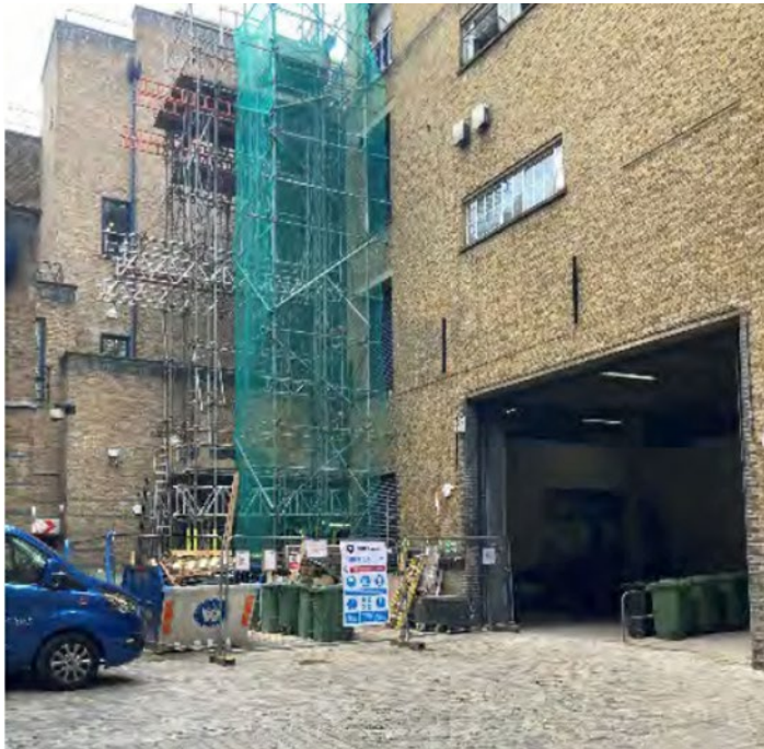
REAR OF 7 LANGLEY STREET (EXISTING)
